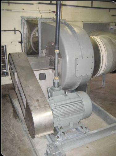
Because the 30-year-old fans were so corroded, it was imperative for their replacements to be highly corrosion resistant. “The existing fans were stainless steel,” said Beyersdorf. “The process was corroding them. They were being eaten away.”
